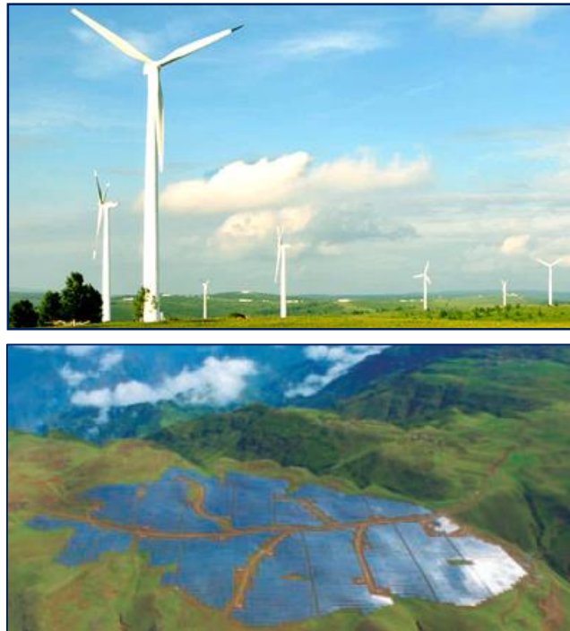
Wind farms/photovoltaic power
